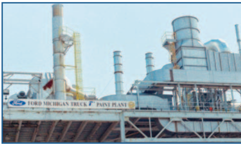
A "Fumes-to-Fuel" installation at Ford's Michigan Truck Plant in Wayne, Michigan. As contaminated process air passes through the fluidized bed's absorber, it is cleaned of its VOCs by the absorption media. When saturated, this media is transported to the desorber, where it is stripped of VOCs by heating it and passing a low volume of carrier gas through it. The resulting mixture of carrier gas and concentrated VOCs is then used directly as fuel in a Stirling engine to make electricity.
